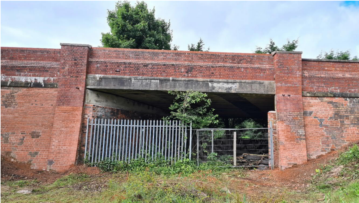
Duddlestone Road Railway Bridge – Extensive brickwork repairs
